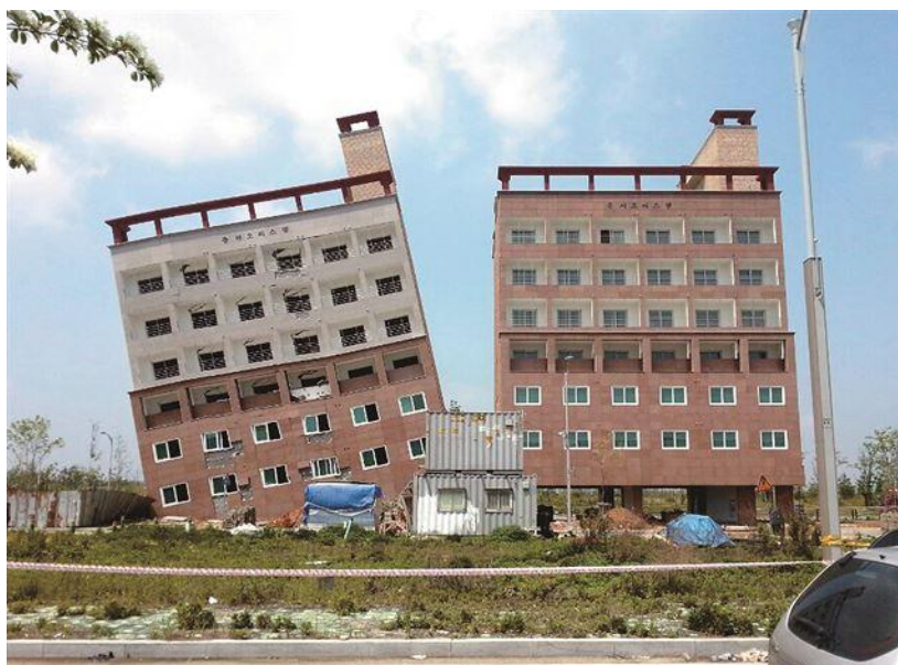
Figure 1. Loss of stability of a residential building in Seoul, South Korea, 2014
