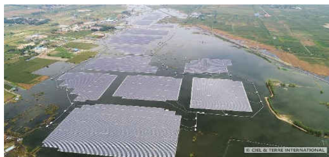
Fig. 4 The 70 MW project
