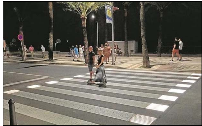
Figure 3. Smart pedestrian crossing.
