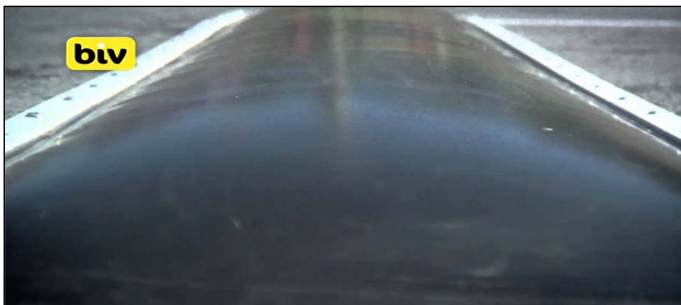
Figure 13. Badenova artificial road roughness.
