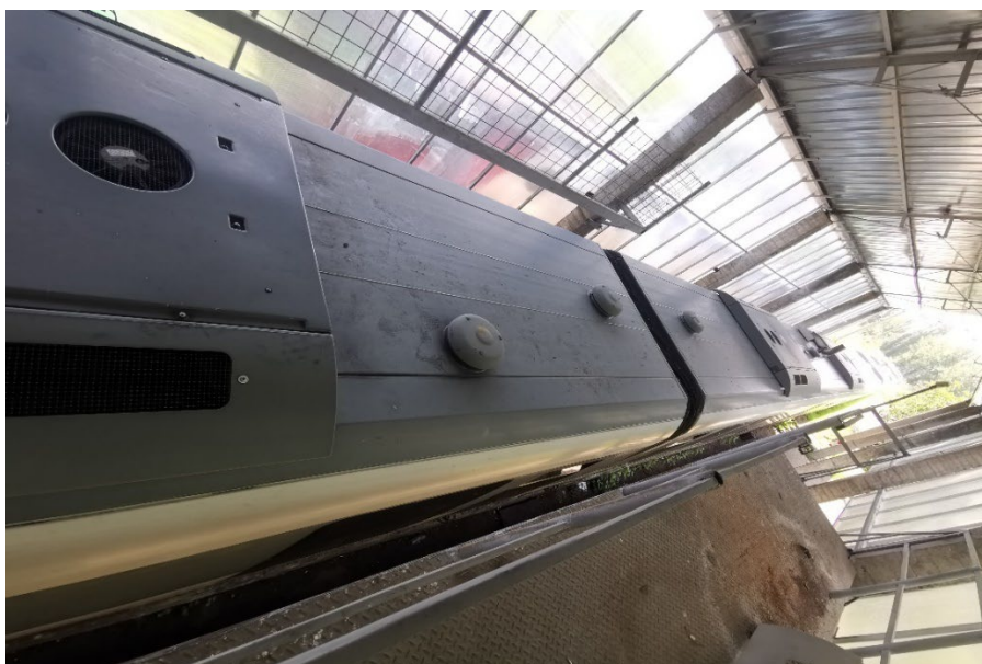
Fig. 9. View with the surfaces available for the placement of solar panels
