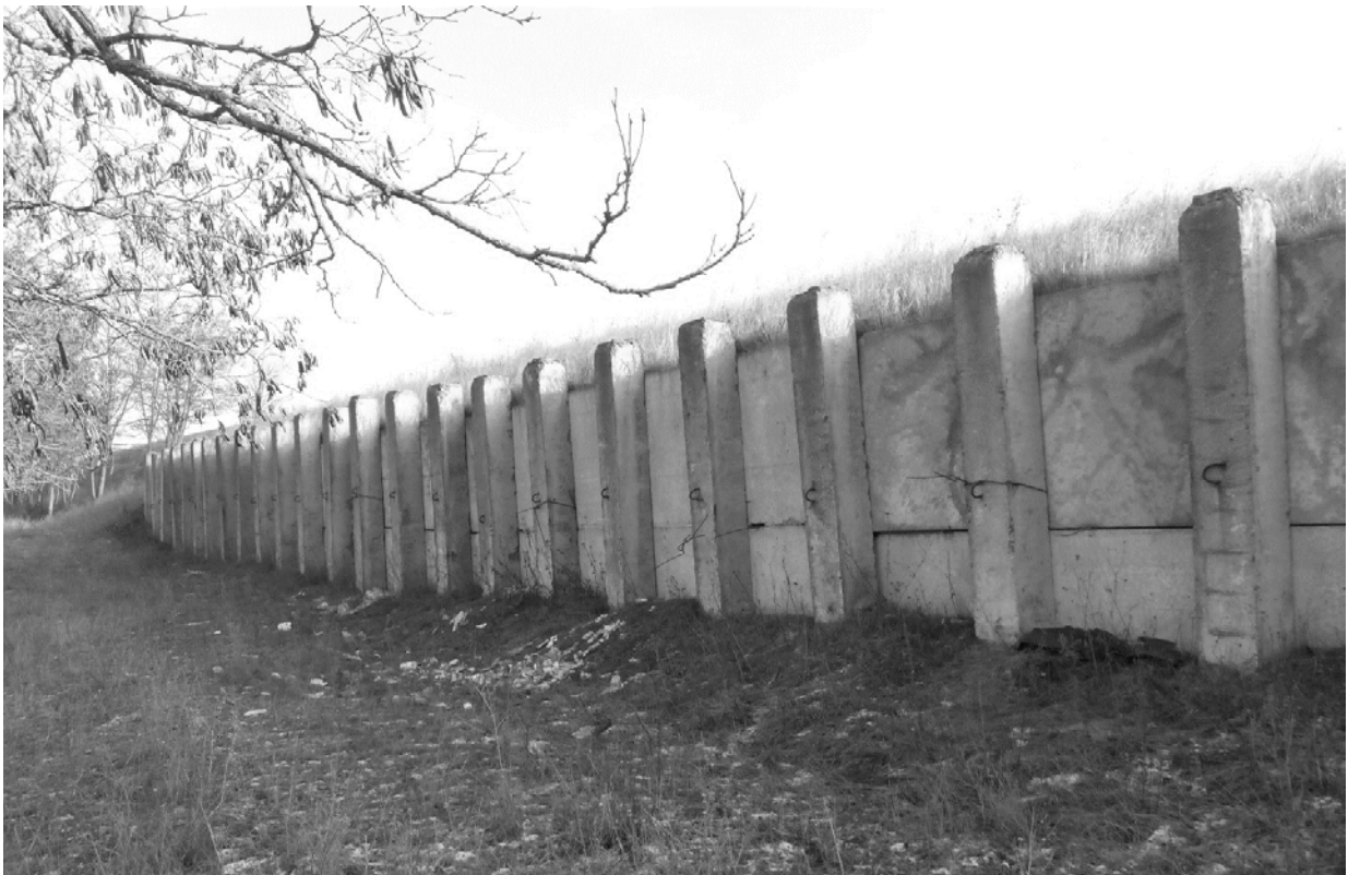
Figure 4. Section of embankment in December of 2019.
