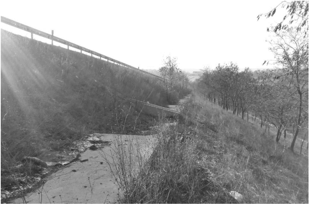
Figure 3. Section of embankment in December of 2019.
