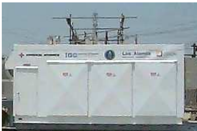
The General Atomics/Intermagnetics General superconducting Fault Current Controller, employing HTS superconductors.
