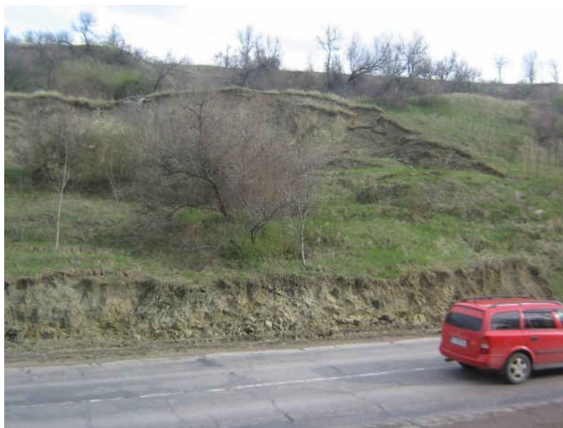
Figure 1. Landslide processes along the M21 road, Brest-Chisinau-Poltava Foto: Polcanov Vladimir, May 2015.
