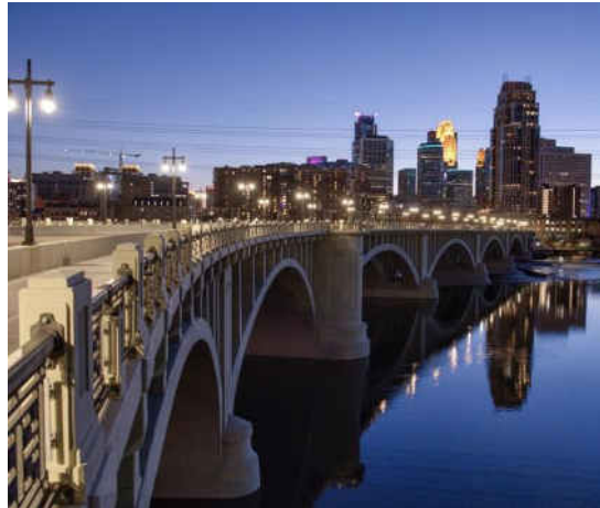
Figura 3. Podul Third Avenue, Minneapolis, Minnesota
